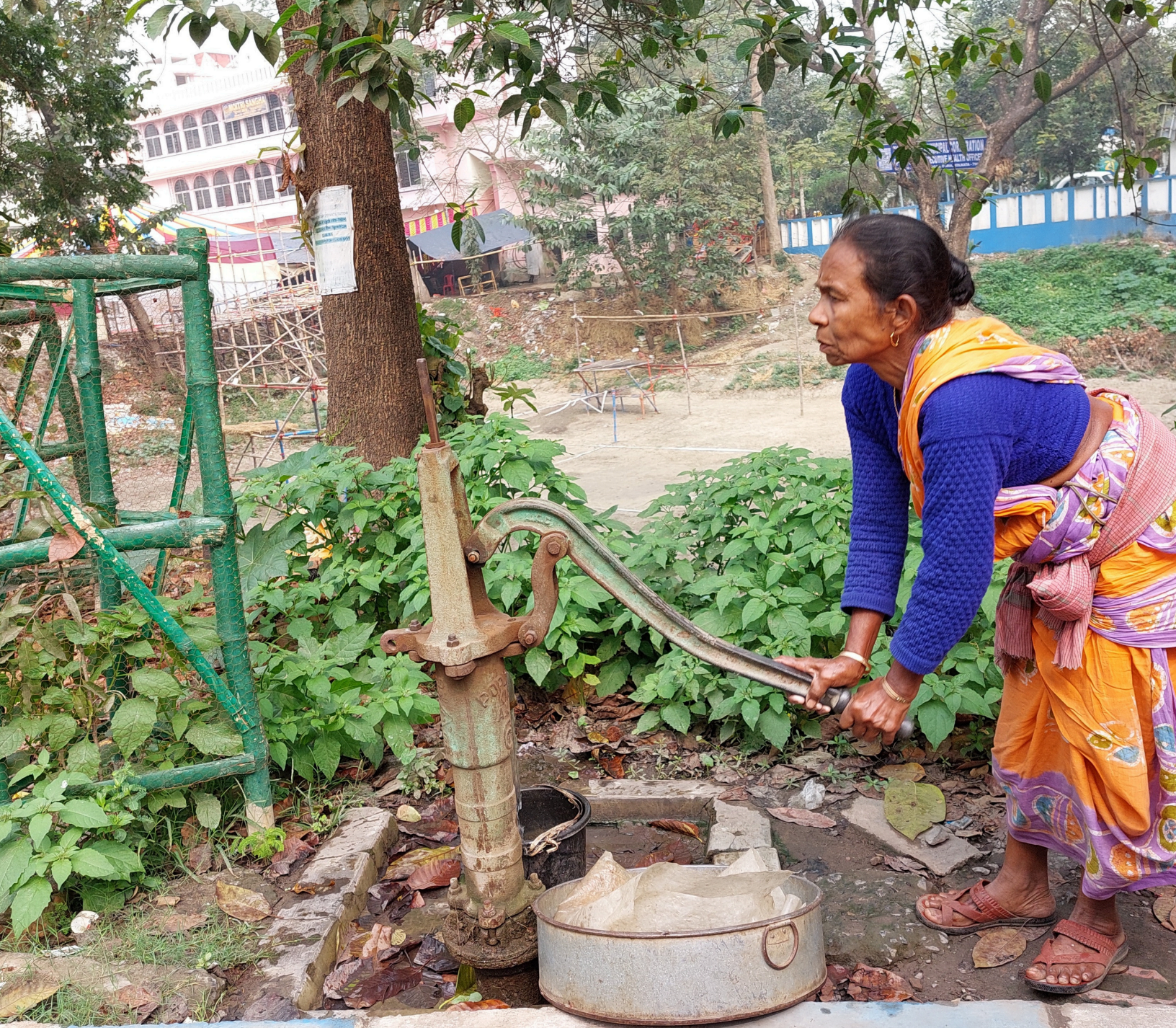
Handpumps accessing shallow aquifers, Kolkata; Source: NIUA
