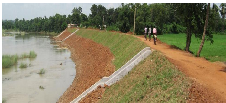
Figure 4- River plain with embankments
