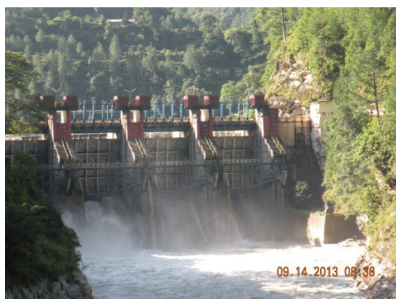
Maneri Bhali-1 Barrage
