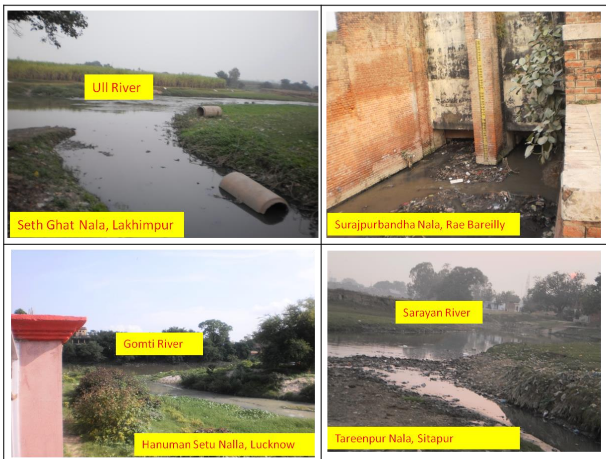
Figure5: Major drains disposing sewage into River Gomati
