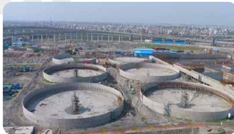
Coronation Pillar- 318MLD STP
