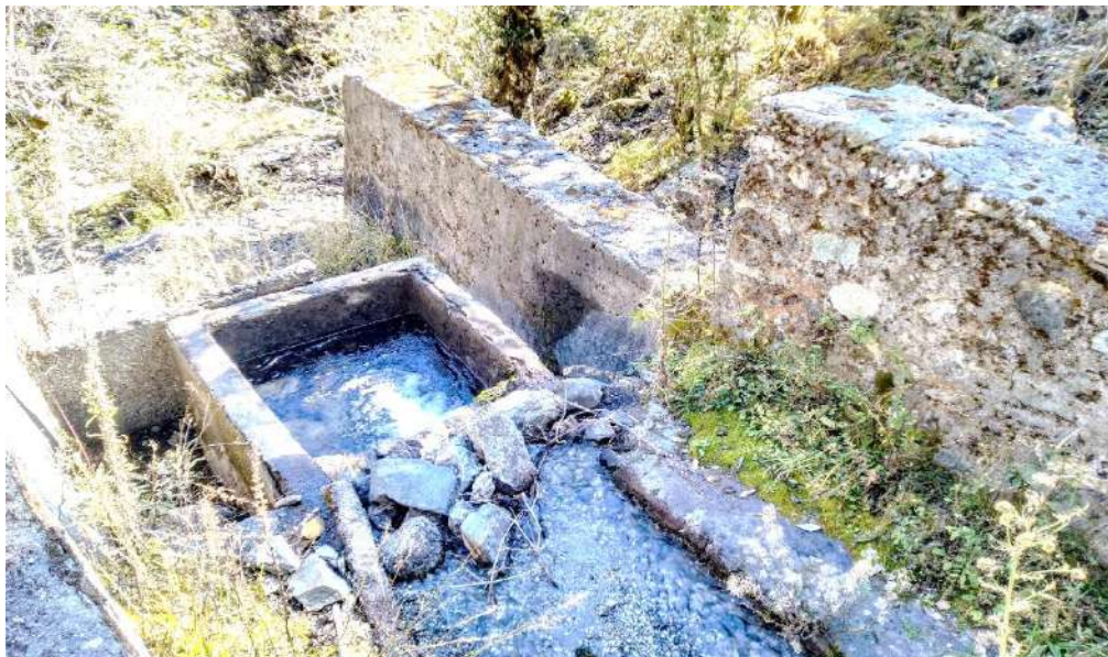
Figure 4.18: Spring water harvesting tank, Taknour Range, Uttarkashi
