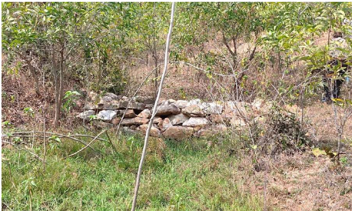
Figure 8.15: Rock check dam constructed in plantation site in Purulia division
