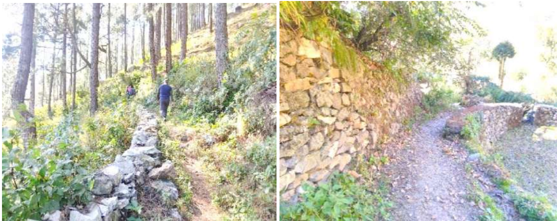
Figure 4.14: Contour bund and retention wall in Uttarkashi Soil Conservation division
