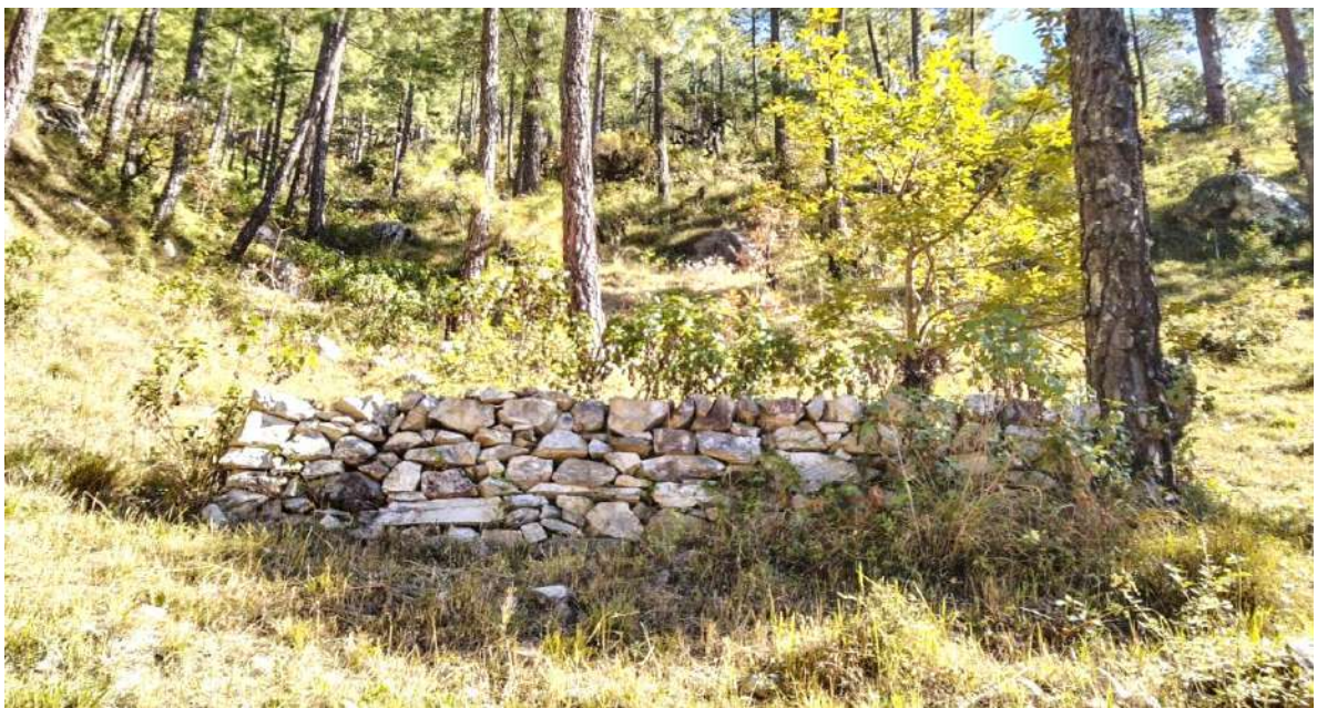
Figure 4.15: Strategic location of gully plug in Uttarkashi division
