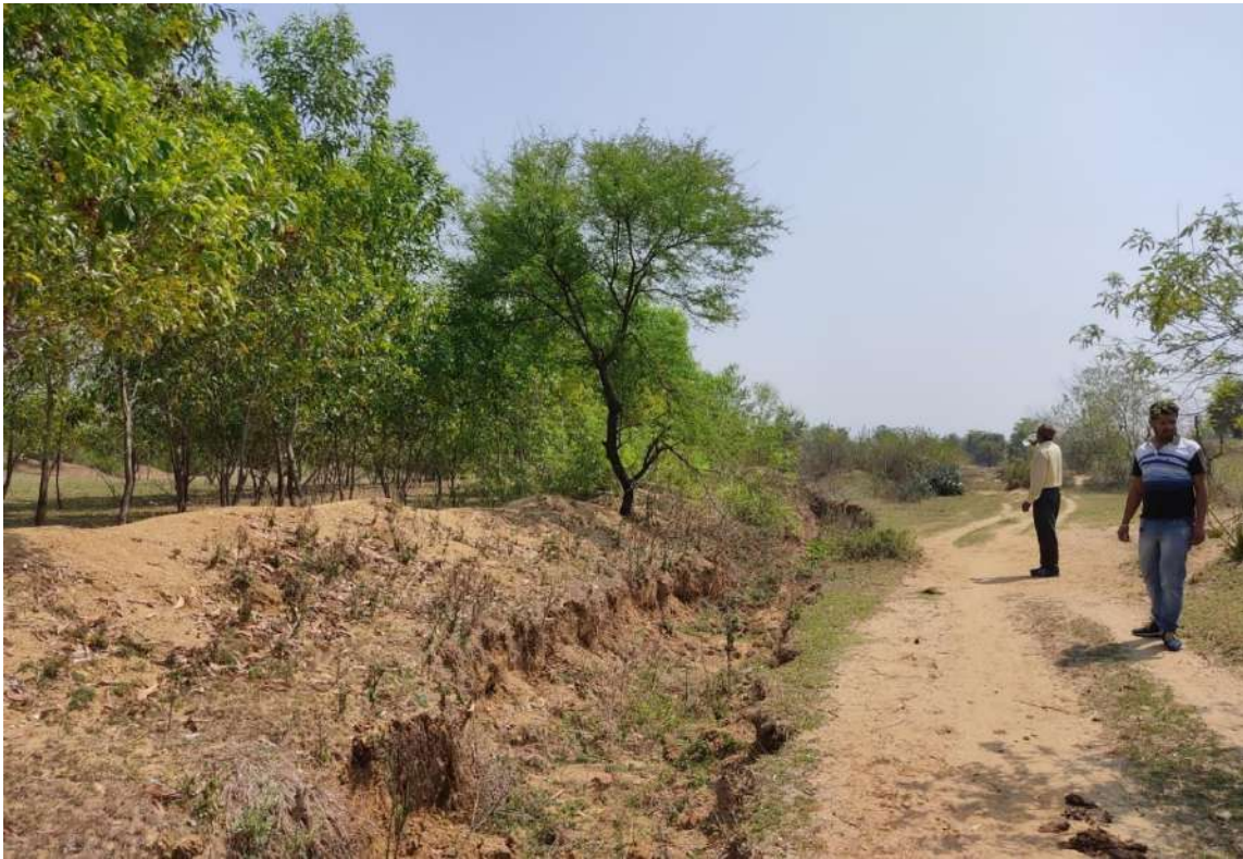
Figure 8.21: CPT is a multi-purpose structure as other than protection from livestock grazing it also helps in site demarcation and arresting surface runoff
