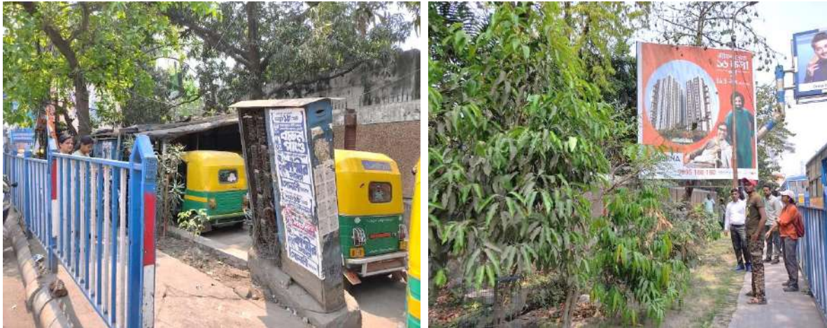
Figure 8.6: Construction of auto stands and erecting hoardings in between the roadside plantations in URF division
